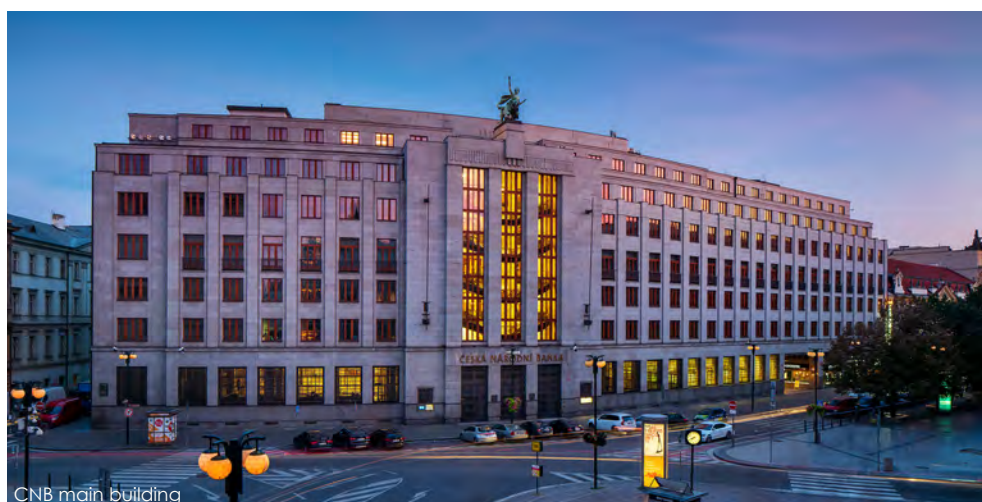
CNB main building
